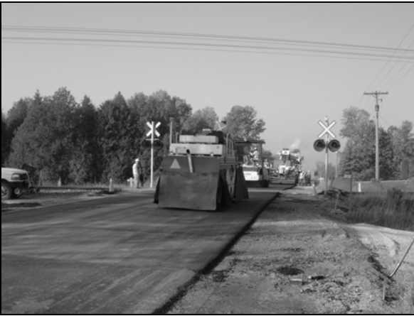
Figure 4c. Intermediate Rolling of Evotherm Mix
