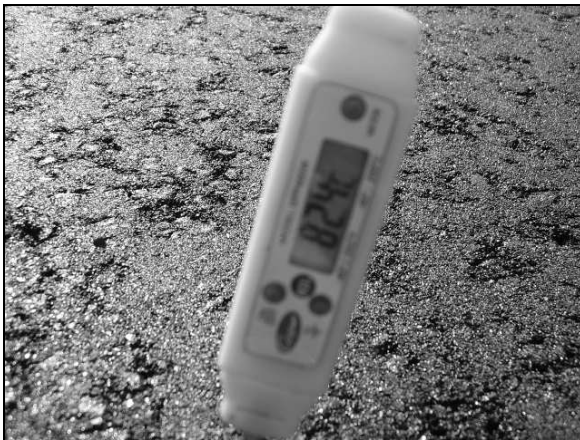
Figure 7a. After Spreader Prior to Rolling
