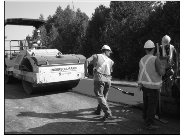
Figure 4d. Rolling the Longitudinal Joint
