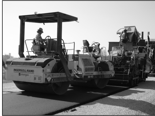
Figure 4b. Vibratory Compaction
