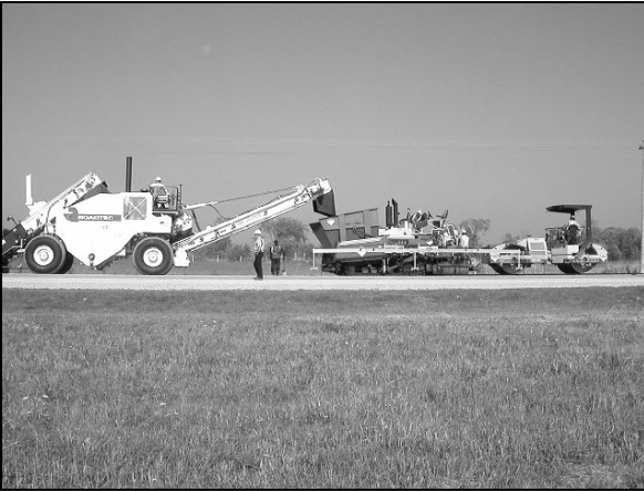
Figure 4a. Placement of Evotherm Mix
