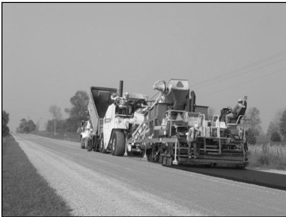
Figure 2a. Laydown with Shuttle Buggy
