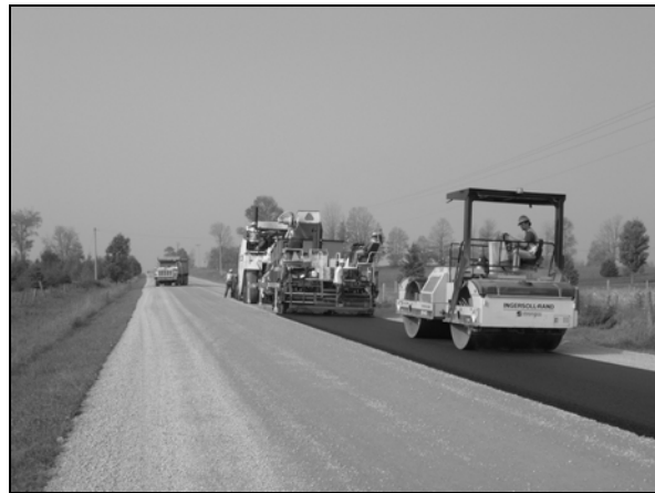
Figure 2b. Vibratory Breakdown Rolling
